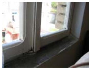
Photo 5. View of a Wooden Frame & Single Glazed Window - Before the EE Interventions
