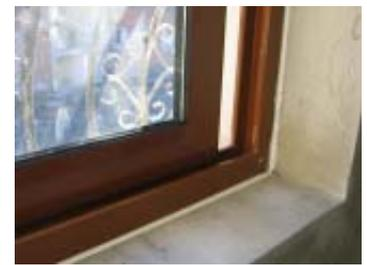
Photo 6. View of a Aluminium Frame & Double Glazed Window - After the EE Interventions
