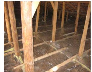
Photo 2. View of Thermal Insulated Roof - After EE Interventions
