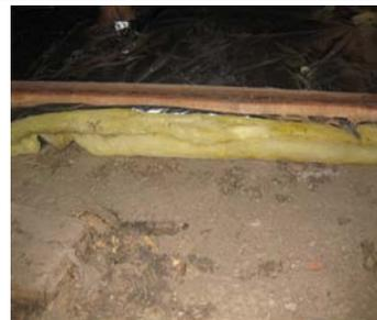
Photo 1. View of Thermal Insulation Works of the Roof - During EE Interventions
